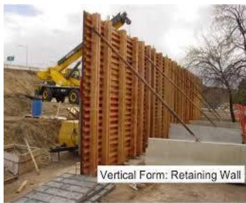
Fig no.7 Wall Formwork
